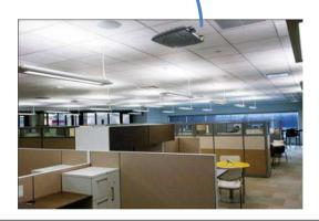
Both rooms/areas with own antenna. The basic package includes 20m RG58 antenna cable. With ECOFLEX cable you can have up to 80m cable length from antenna.
